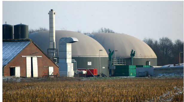
Vergistingsinstallaties (Bioelectricitalia & Rtdvrenthe)
